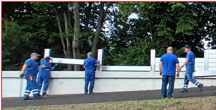
Installation of linear protection
