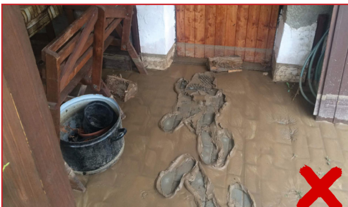
Before installation of the system
