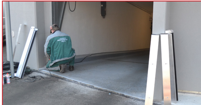
Installation of lateral guidances
